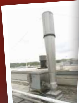
Venturi Exhauster at Fresh Mark's Salem, Ohio plant
