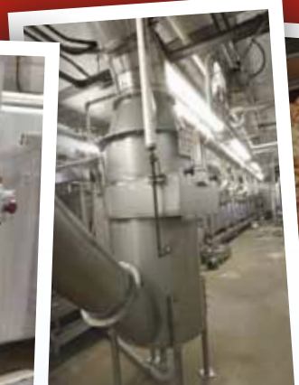
Demister Filtration Unit
