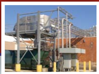
The blowers, separator, and compactor of Dietz & Watson's casing removal system are located outdoors.
